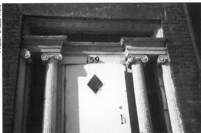
Transom detail of the carved woodwork in the Greek Revival entryway.
