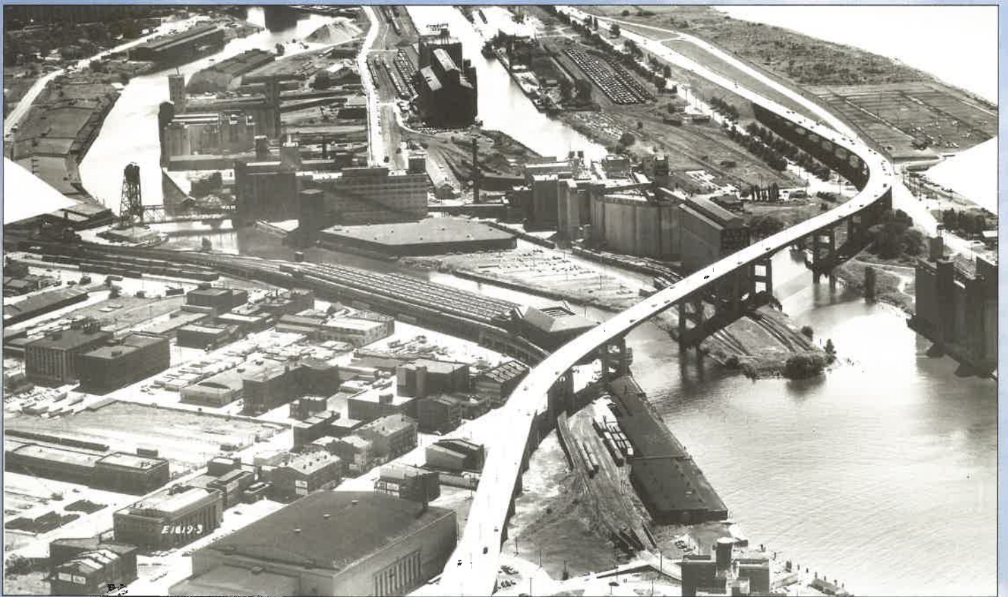
A southerly view of Buffalo Harbor and the lakeshore from the late 1950s. Several 1830s-vintage buildings still remain on lower Main Street, as does the Lehigh Valley Terminal, across from the Aud. This image clearly shows the Skyway turning to avoid the famous, now demolished, Dakota elevator with the "Gold Medal Flour" sign (right center). WESTERN NEW YORK HERITAGE PRESS
