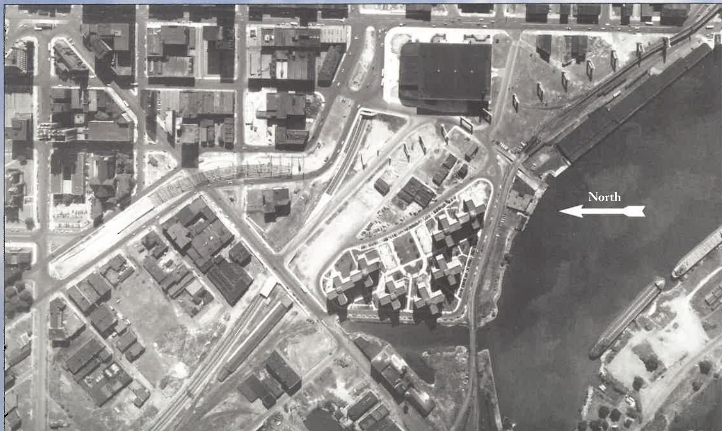
Construction begins – In this aerial view from July 1954, the concrete pylons have been raised for the Skyway's path around Buffalo Memorial Auditorium (center) and work has begun on the northern approach ramp paralleling Terrace and Franklin streets.
