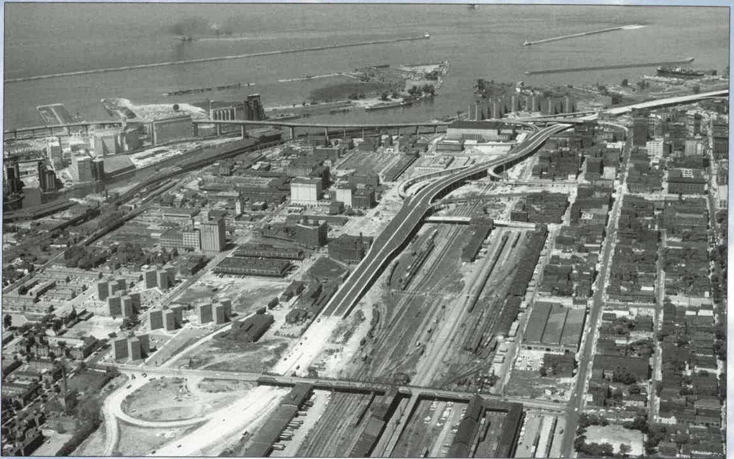
A "ribbon of steel and concrete." These two panoramic views from the early 1960s track the Skyway's route across Buffalo's harbor entrance. Note the progress being made on the Niagara Section of the New York State Thruway (I-190) in the center of both images, where the paved section is nearing what will become the Louisiana Street exit. WESTERN NEW YORK HERITAGE PRESS
