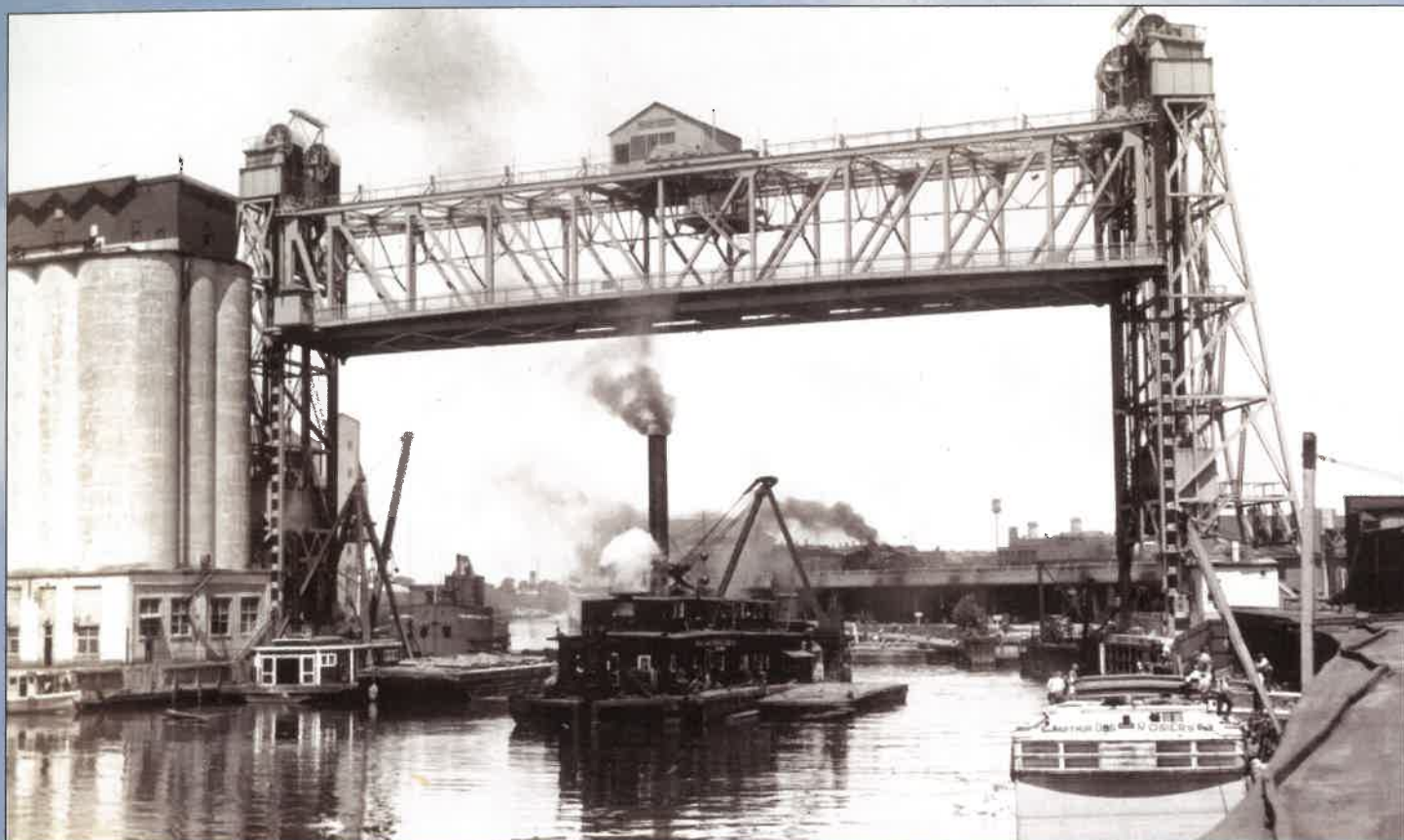
A view of the Michigan Avenue lift bridge, prior to 1939. The need to raise the bridges to allow ships in and out of the harbor was the cause of "almost daily, serious jams" for traffic traveling between the city and the southern lakeshore. In this image, a dredging boat is passing underneath the bridge while a canal boat is tied up at right.
