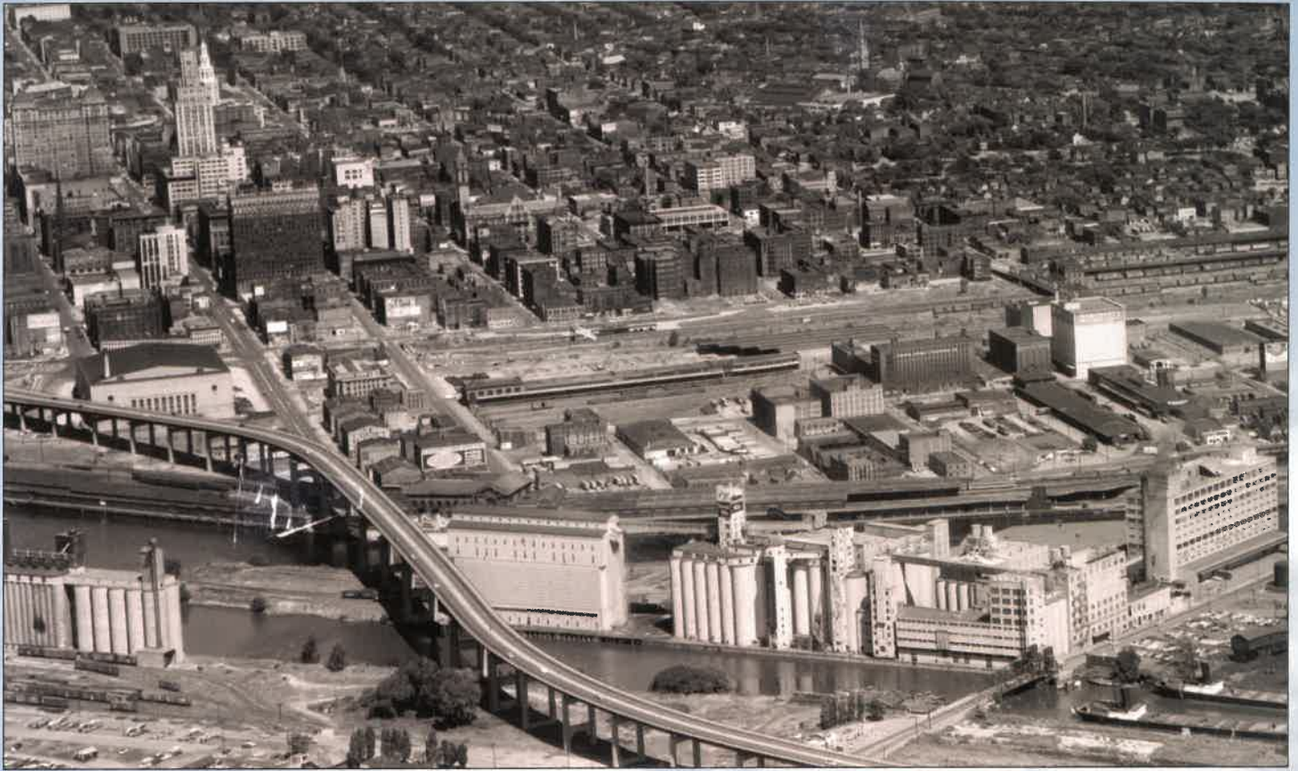
The old and the new – The Michigan Avenue bridge over the City Ship Canal in the right foreground is dwarfed by the new, modern Skyway in this view from the mid-1950s. WESTERN NEW YORK HERITAGE PRESS
